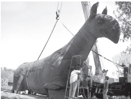
Baluchitherium model being installed.
